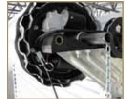
Insulation is made of a foil backed, dual layer of heavy-duty polyethylene air-bubble insulation secured in place with a strong adhesive and joined by mylar film to provide an R value of 4. (Top draft stop and side draft stops are also included.)
